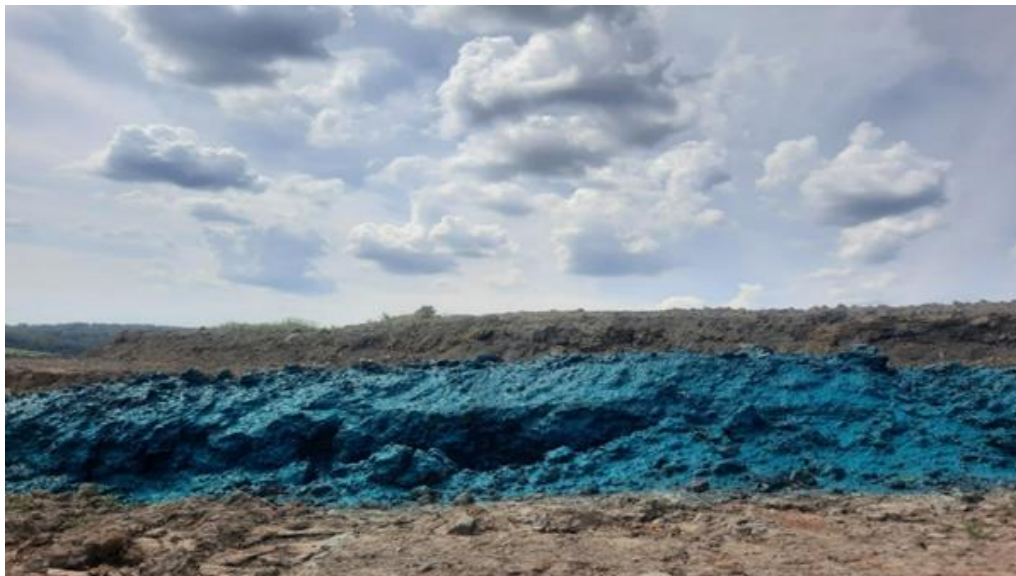
Figure 2: The site after the hydraulic seeding works
